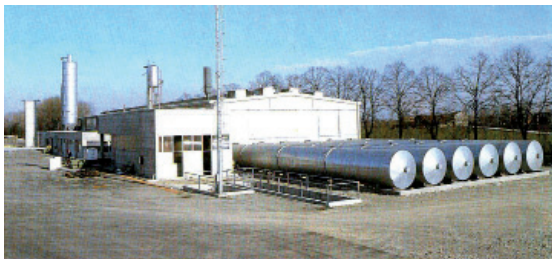
Hebel plant of 1986
