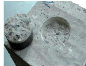
Fig. 14. Cohesive failure of concrete adherend
