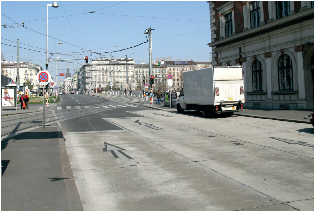
Fig. 13. Visual impression of a concrete paved holding range in Vienna in 2007; 3-4 years after placing. Directly before and directly after the pictured holding range the pavement is made of asphalt.
